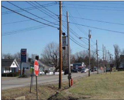
Overhead utilities, drainage, no sidewalk
