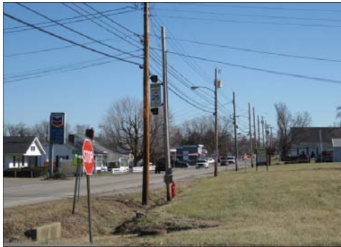
Existing Above Ground Utilities
