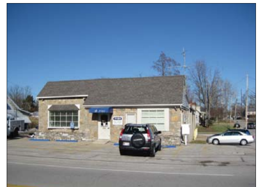
West Shelby Water District Office
