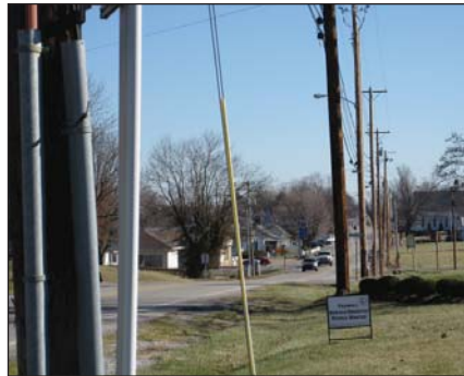
No sidewalk, overhead utilities
