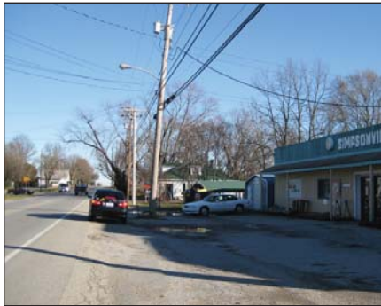
Unrestricted access, outdoor storage, overhead utilities
