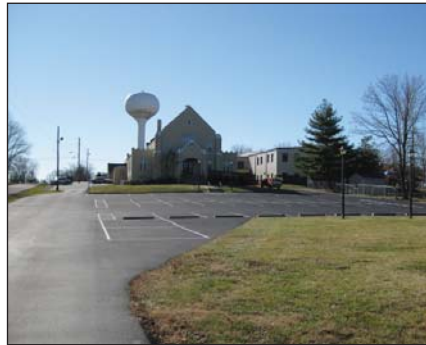
Large parking area fronts US 60
