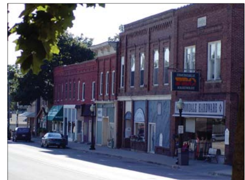
District Identity Exercise - Village Branding
