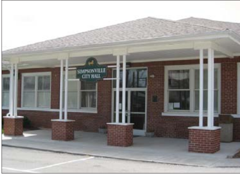
City Hall on Old Veechdale Road
